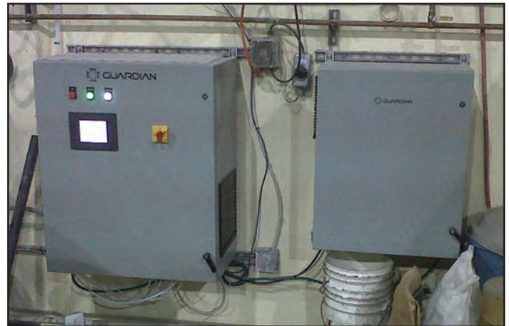
Original ozone system has now been replaced by a system from the same manufacturer to provide for 120 g/hr, which is giving the plant twice the ozone at lower power consumption.
