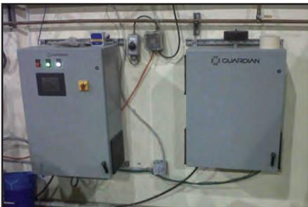
The system consists of one box including the ozone generators and most of the electronic controls, and another box for the oxygen concentrator, the rest of the electronics, and other equipment. The only maintenance required is to clean the incoming air filters daily, which is accomplished in five minutes or less with a simple compressed air blow-out.
