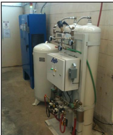
Installation of replacement ozone system allowed for assurance of sufficient ozone delivery to tunnel washers, while providing new levels of diagnostics and control to help management optimize quality and efficiency. In addition, the plant has benefitted significantly from a much smaller footprint for the new system.
